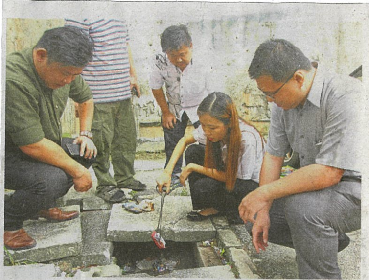
Heng (second from right) showing a clogged drain at the Taman Midah low-cost flats in Cheras, Kuala Lumpur.
