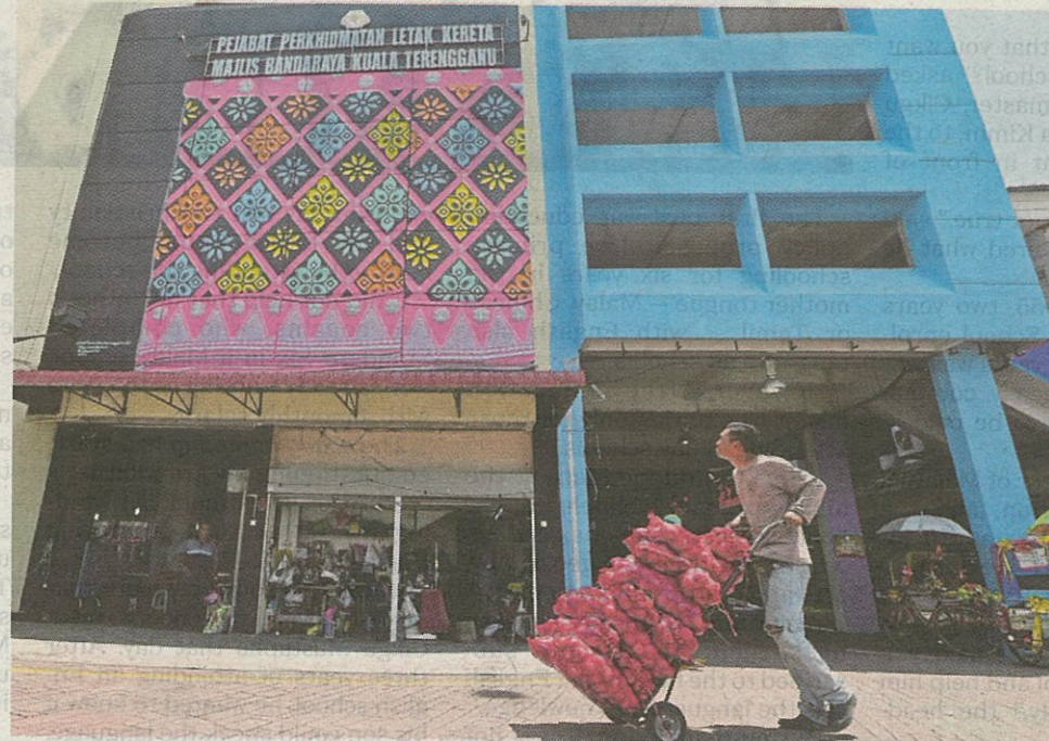
Two months ago, the building's exterior was painted in vivid colours and decorated with batik and songket murals for Hari Raya Aidilfitri. PIC BY GHAZALI KORI
