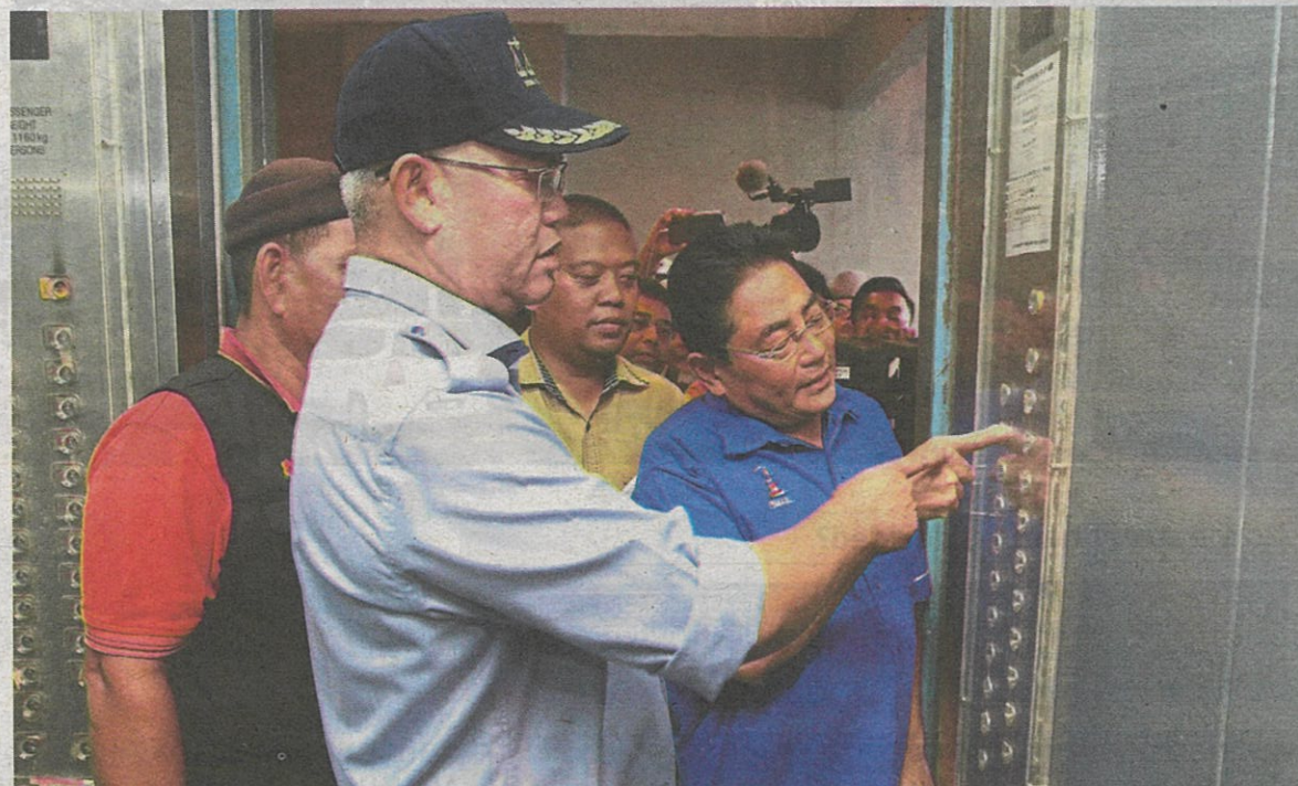
Noh (in cap) discussing with Ampang Umno division chief Datuk Ismail Kijo on the need to repair a faulty lift at Taman Industri Flats in Lembah Jaya, Ampang.
