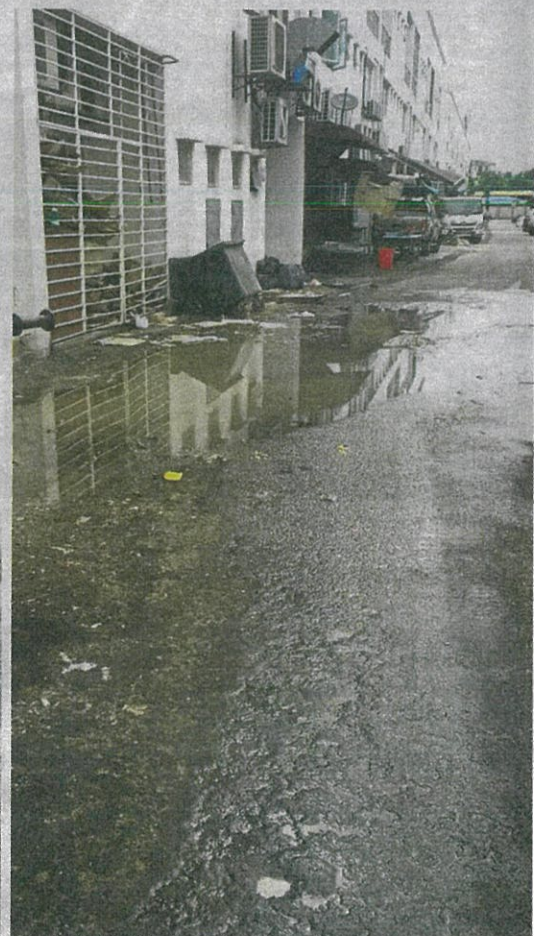
This backlane is waterlogged with wastewater that overflowed from clogged drains.
