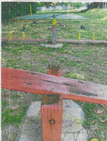
Potential danger: A see-saw with a protruding metal stand is a safety hazard for visitors to this public park.
