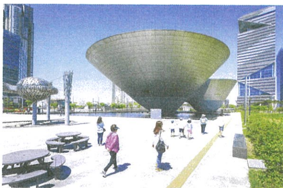
Tribowl Building at Central Park in Songdo, South Korea
