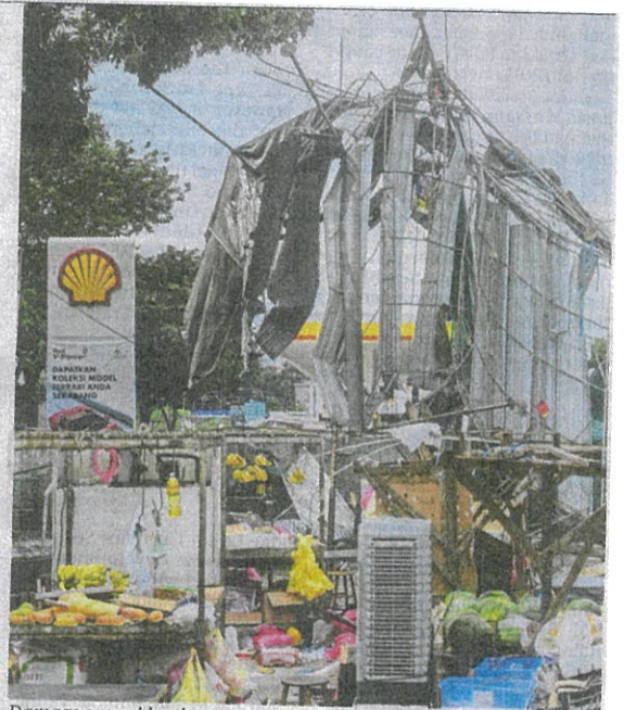
Damage caused by the storm on Friday in George Town. FILE PIC
