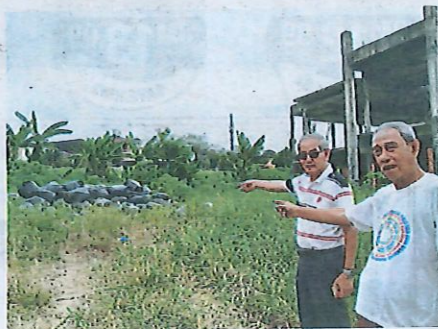
Safety risk: Chang and Ahadde pointing to the abandoned construction site in Gertak Merah.
