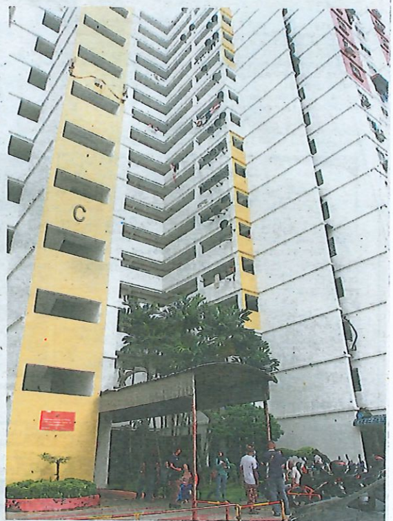
Incidents like the lift that crashed in PPR Kerinchi, Kuala Lumpur, show how important it is for everyone to take care of the facility in their buildings. — Filepic
