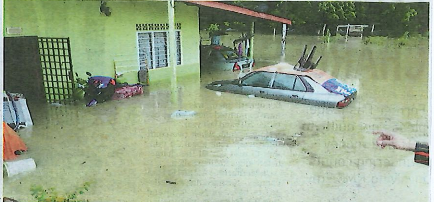
Faulty drainage systems caused several houses to be flooded after heavy rain at Jalan Lurah 19, Kempas Baru, Johor Baru, yesterday. PICTURE COURTESY OF FIRE AND RESCUE DEPARTMENT
