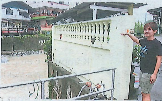
Resident Teoh Jen Mei, who lives beside the river, showing how high the water rose to during the Oct 9 flash flood in Kampung Cempaka.
